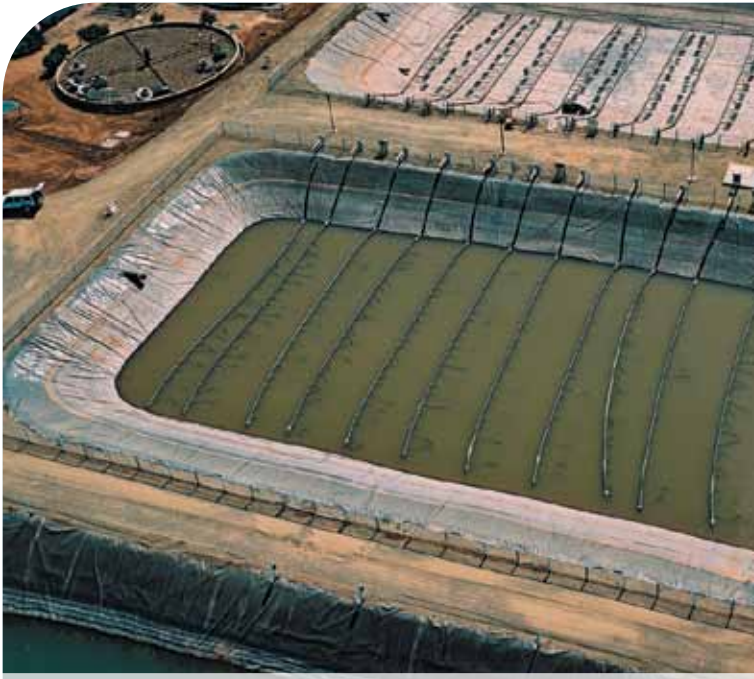
Biolac® basins with rectangular, flat bottom clarifiers
