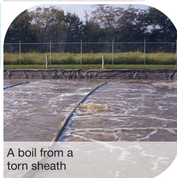
Air leak in the previous style float
