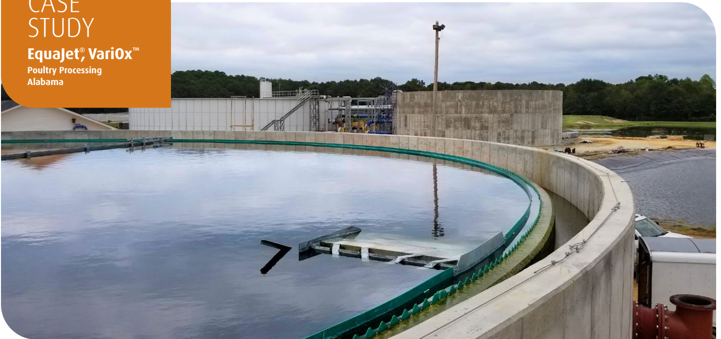
Secondary clarifier with nitrification and anoxic basins in background
