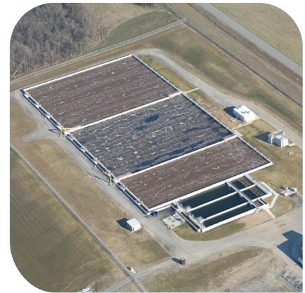
the winter of 2006/2007. It has consistently met the 50 mg/l BOD discharge limit that was required, and the treated effluent is now directly discharged into nearby Gunpowder Creek, without adverse effects on the environment.
