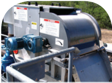
Screens discrete solids, scum and oily materials without blinding
